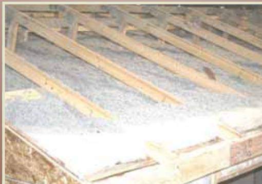
**Blown insulation eliminates gaps in the roof insulation and lowers energy costs.**
