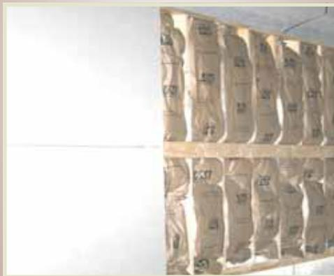
**Pre Notched exterior wall studs reinforced with 1x6 at the drywall seam create horizontal joint support to help reduce cracking and produce a stronger sidewall.**
