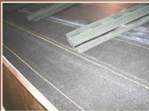
Ice and water shield installed over ply dry roof sheathing helps eliminate any water entering the roof cavity and is effective against any potential ice buildup.
