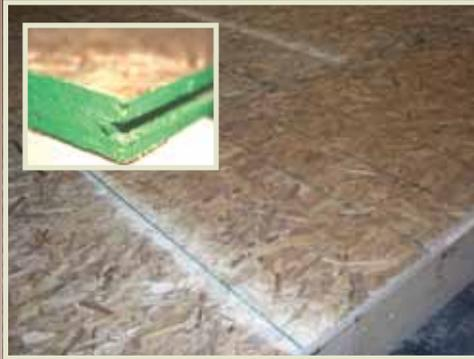
**3/4" tongue & groove O.S.B. floor is one of the strongest most durable decking materials available and it creates an even floor.**
